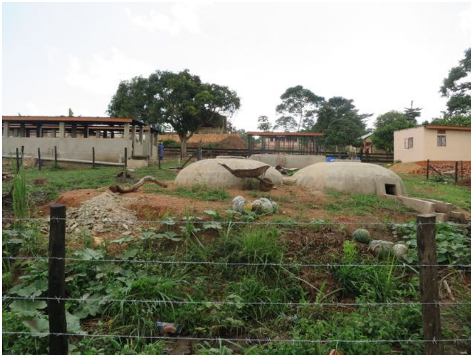
The bio-digester system at KPVS
