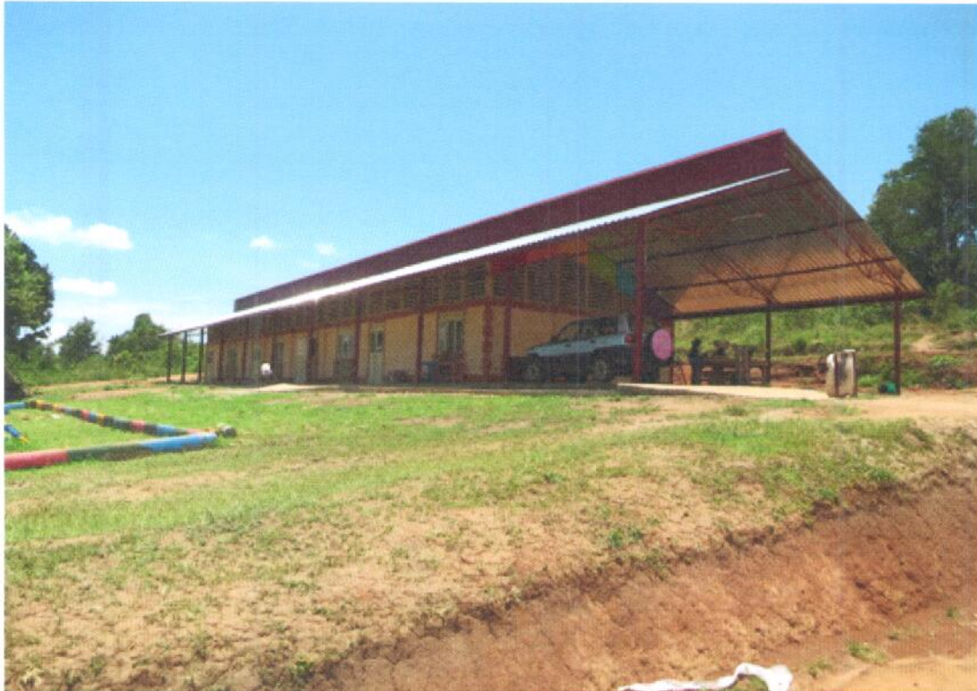
ECD, Assembly Hall and Tailoring centre complete at Katuuso.
